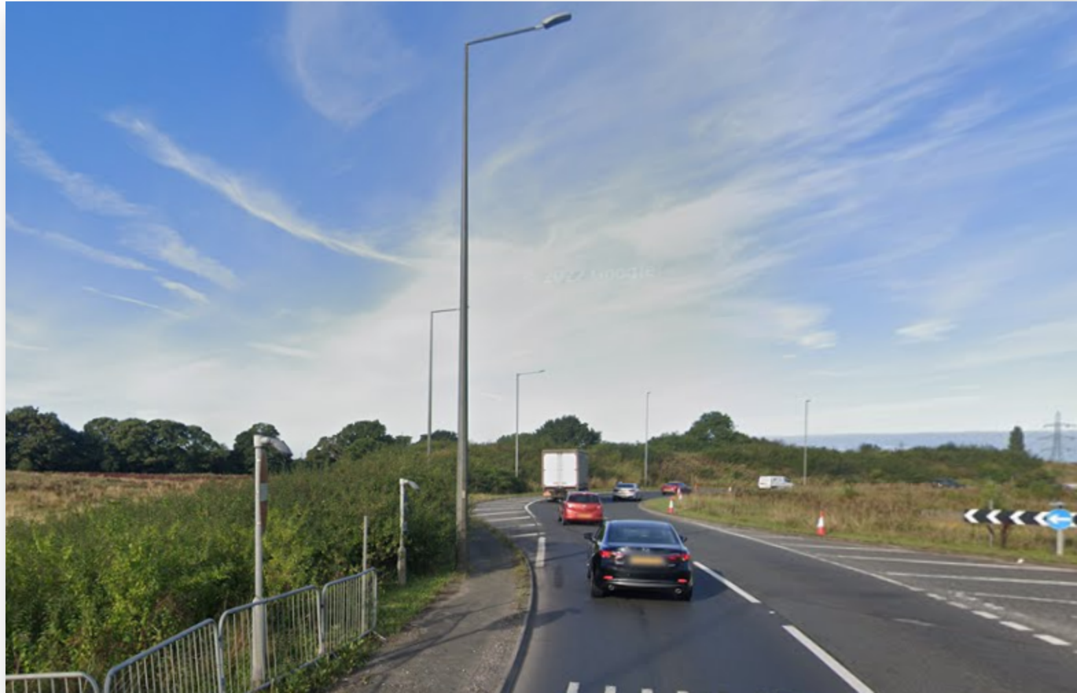
Approach to the M65 terminus roundabout
