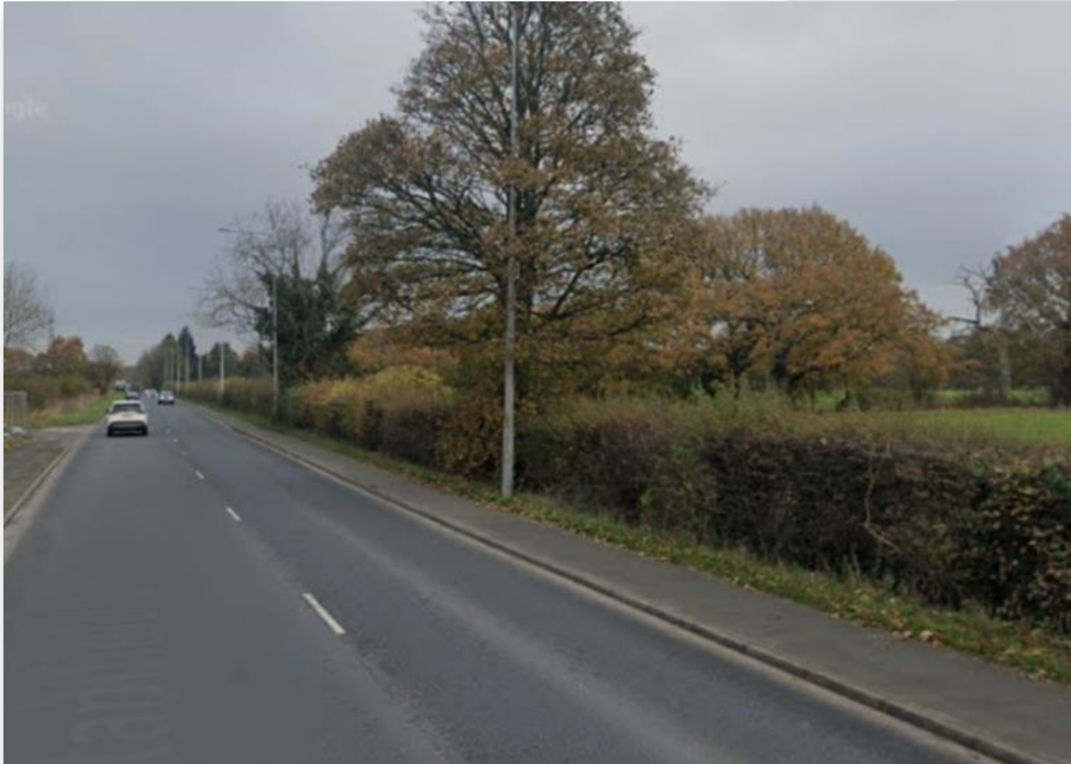
Stanifield Lane at Zone D
